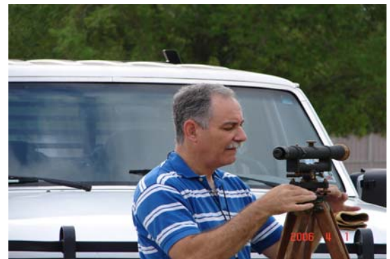
County Extension Director Vince Mannino helps shoot the grade in the Front Yard garden so that the proper slope can be calculated for drainage purposes.
